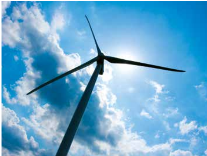
Wind electric power generators
