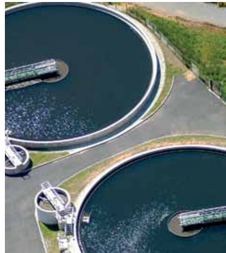
Water treatment facility – a contributor to pollution-based corrosion
